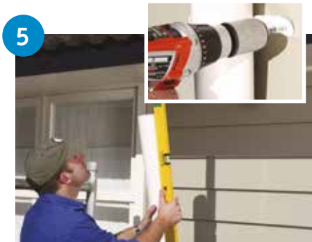
5 Use a level or plumb line to mark where the downpipe will sit against the wall. Ensure downpipe clips are spaced no more than 1.2 metres apart and the first clip is a maximum of 200mm below the downpipe bend. Downpipe clips to be secured with two stainless steel screws.
