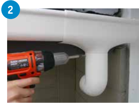
2 Connect downpipe bend to expansion outlet using a screw to hold bend in place. To allow easy removal for cleaning debris do not solvent cement bend to outlet.
