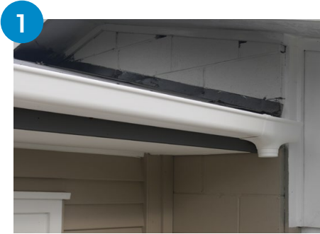
Install expansion outlet as per spouting installation instructions.
