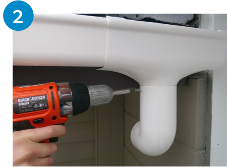
Connect downpipe bend to expansion outlet using a screw to hold bend in place. To allow easy removal for cleaning debris do not solvent cement bend to outlet.
