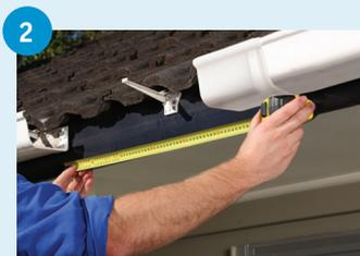
Replace any damaged brackets. Place joiner and expansion joiner then measure distance in between for replacement piece.
