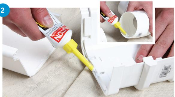
Marley solvent cement (MCS®) should be applied evenly to **both surfaces** being joined. Then press both surfaces together and hold for 20-30 seconds
