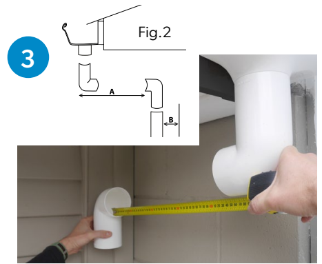
Determine the offset length (A) using Fig 2 allowing for depth of socket and taking into consideration the downpipe bracket distance from the wall (B). Cut downpipe as per measurements.
