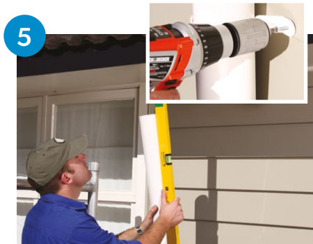
5 Use a level of plumb line to mark where the downpipe will sit against the wall. Ensure downpipe clips are spaced no more than 1.2 metres apart and the first clip is a maximum of 200mm below the downpipe bend. Downpipe clips to be secured with two stainless steel screws.
